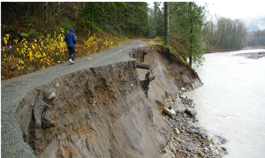
The Suiattle Road is washed out in several locations, with the most severe removing entire sections of pavement. Photo by Kim Brown
