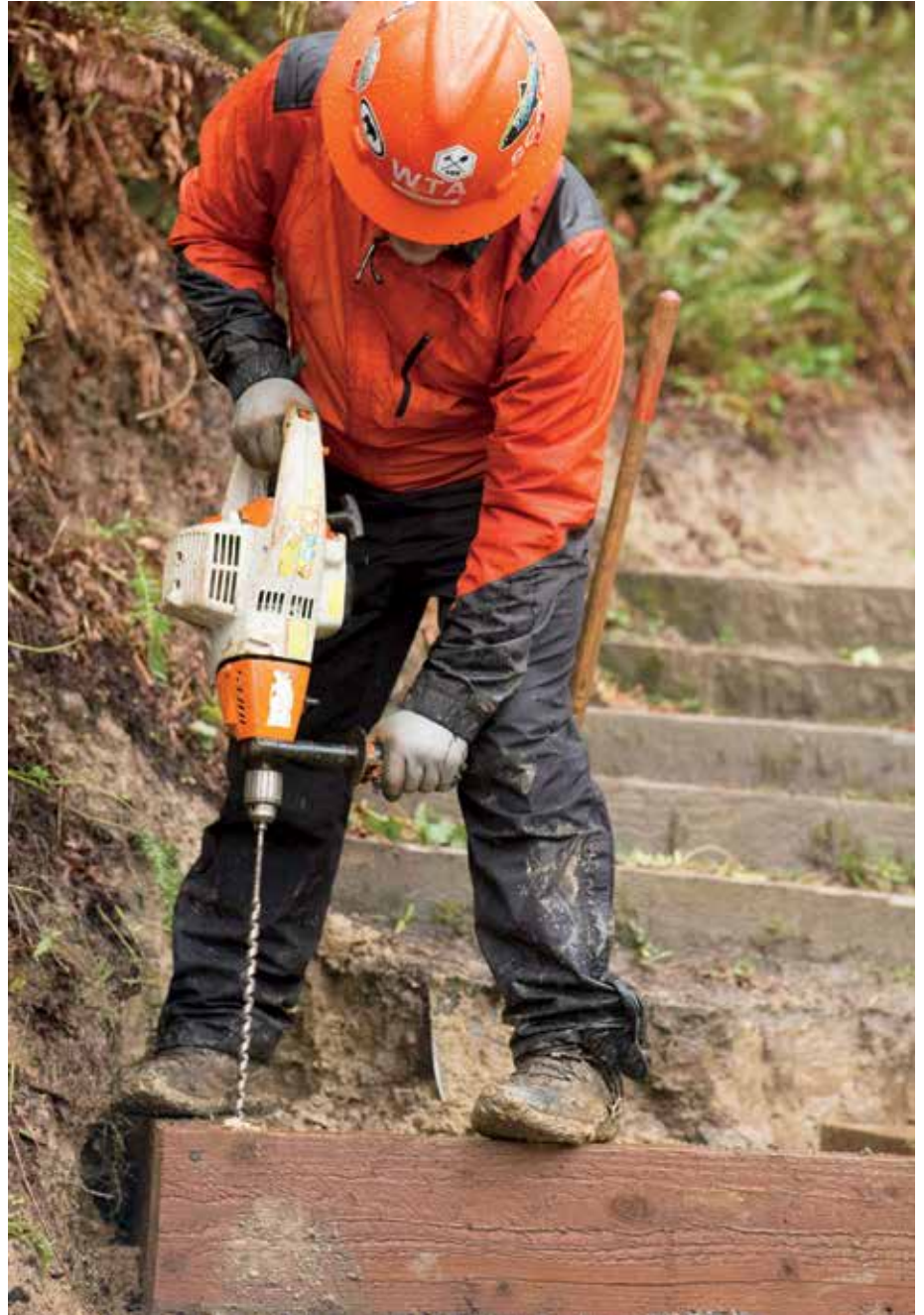
At top: Volunteers built 86 new steps at Meadowdale Beach Park in Edmonds. Photo by Barbara Ingram. Above: At Priest Point Park in Olympia, crews worked on a set of steps that lead down to the beach. The work involved power tools, which is unusual on WTA work parties. Photo by Emma Cassidy.
