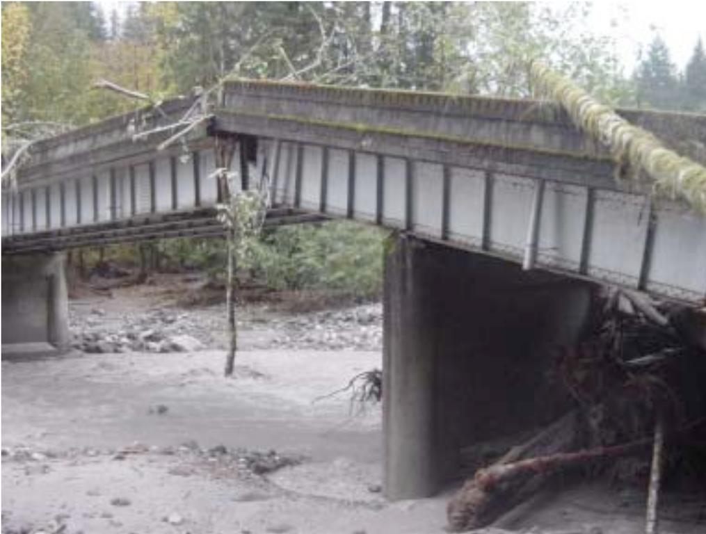
*Forest Service roads were also hard hit. This bridge on Whitechuck River Road #23 was demolished during an unusually warm October rainstorm. The road, which has been shut down indefinitely, leads to such popular areas as Kennedy Hot Springs (which is now buried beneath rock and mud).*
